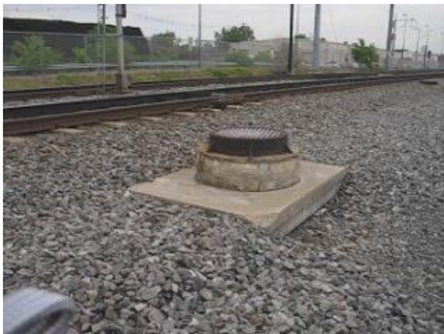
Photo B-12 (Typical System-wide Manhole in ROW)
