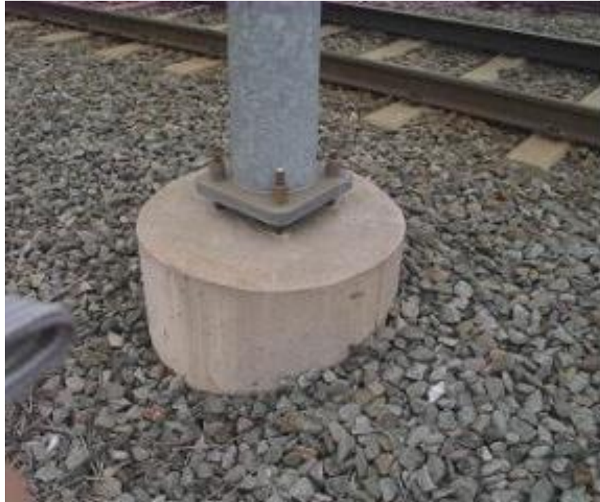
Photo B-11 (Typical Catenary Pole Foundation in ROW)
